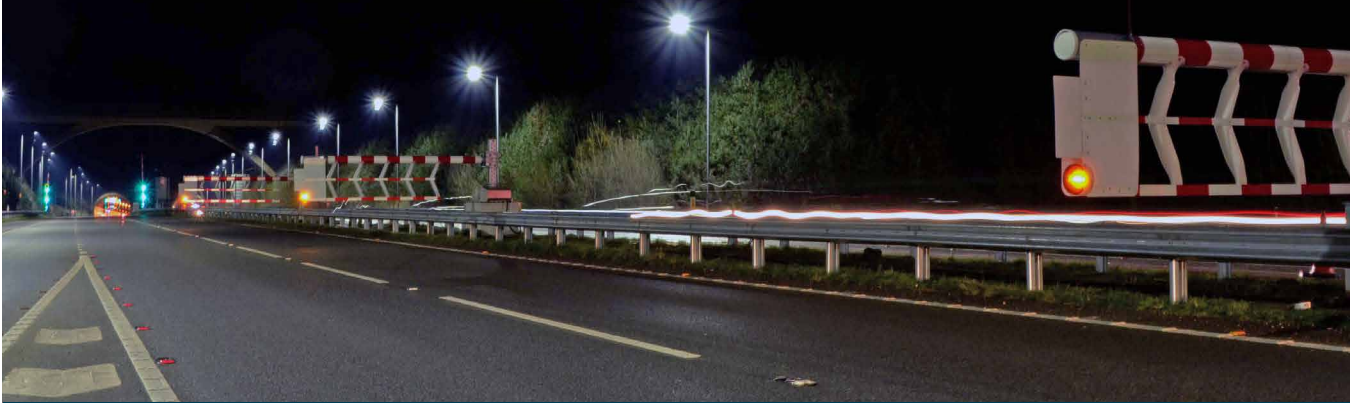
Highway Care's SwiftGate automated taper deployment system in action
